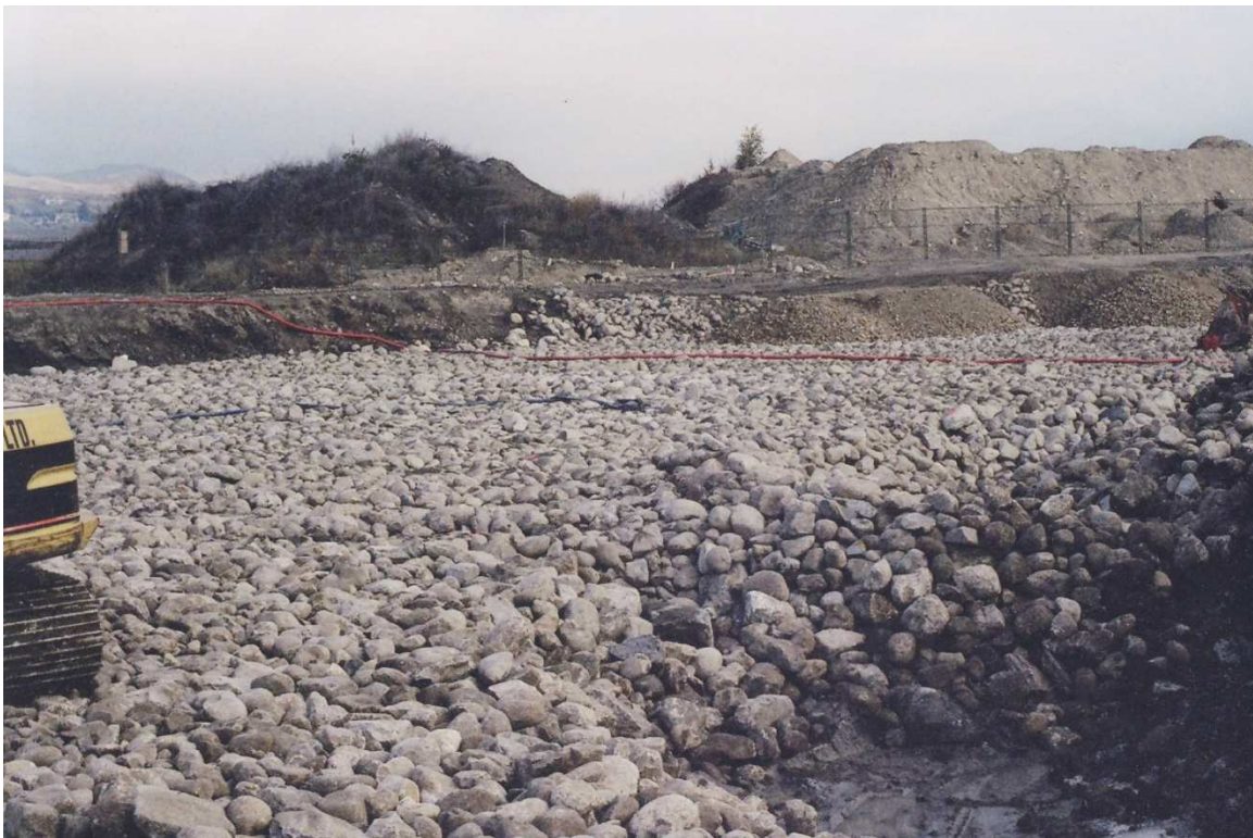
Figure 7 Backfilling the Foundation Excavation
